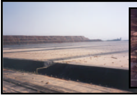
Heap leach pads in Ghana
