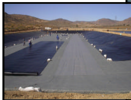
Oxidation ponds at Bergsig
