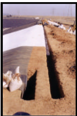
Bentofix installed at Newcastle
