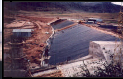
Mafeteng dam wall, Lesotho
