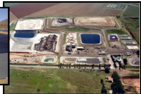
Holfontein Landfill site in Gauteng
