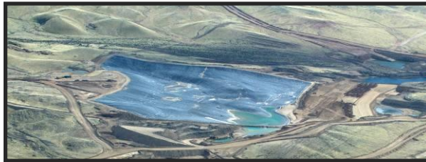
Tailings Storage Facility
